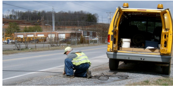
Installing portable traffic collection device
