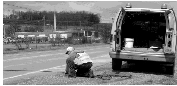
Installing portable traffic collection device
