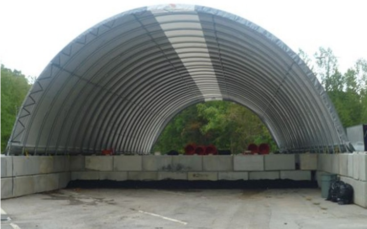
New salt storage facilities will be strategically placed along the Interstate system.
