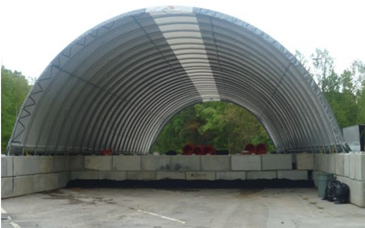
New salt storage facilities will be strategically placed along the Interstate system.
