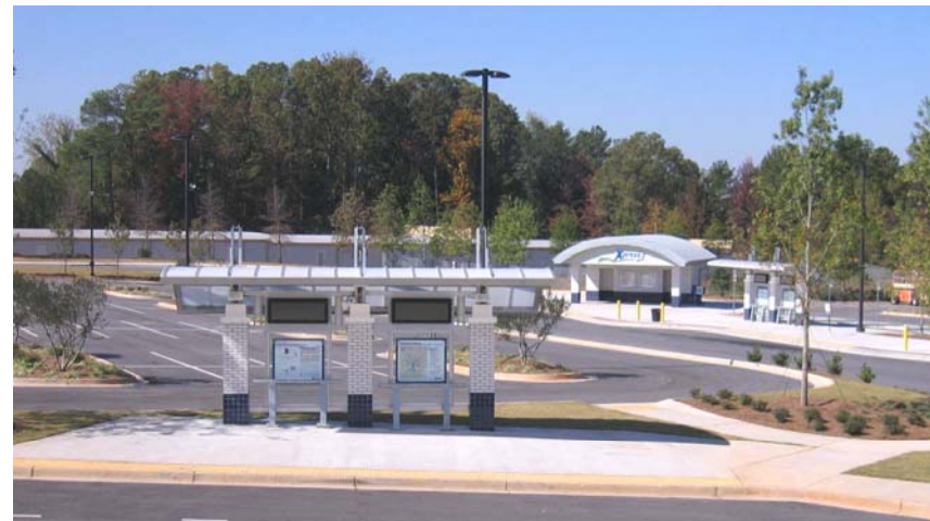
Panola Road Station - Opened April 2007 Capacity - 586 parking spaces October 1, 2008 – 602 cars
